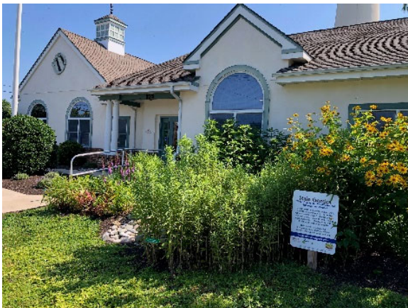
Municipal Building Rain Garden
